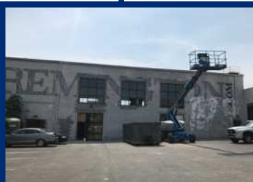
FastForward U Under Construction 2017-2018
